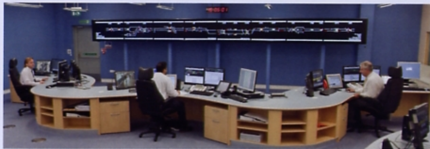
Osborne House control room.
